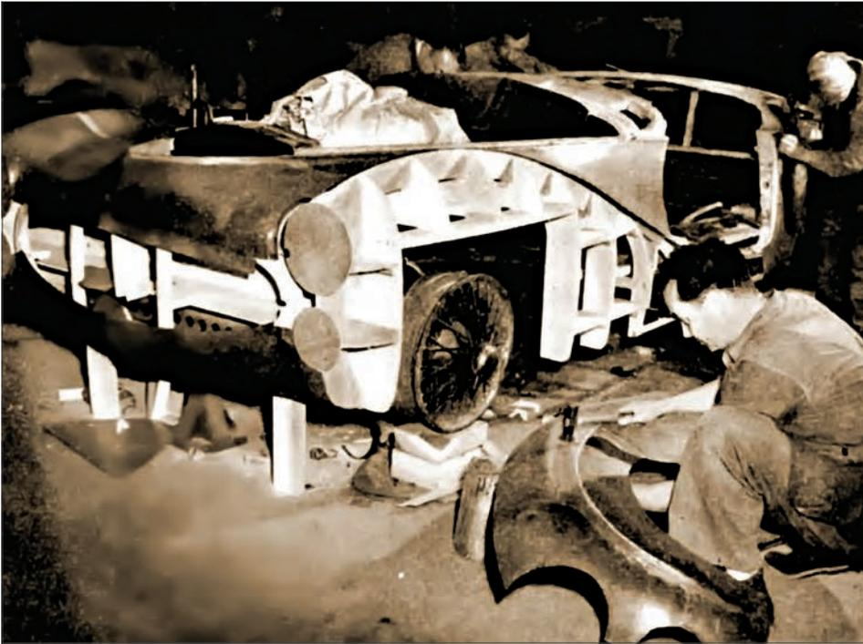
Saoutchik's workers test fitting the outer front fender panel on the wood *maquette*. The cowl and front valence panels are in place and being prepared for welding. (*France Magazine, Peter Larsen*)
